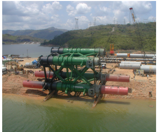
Chiapas Bridge Pile
