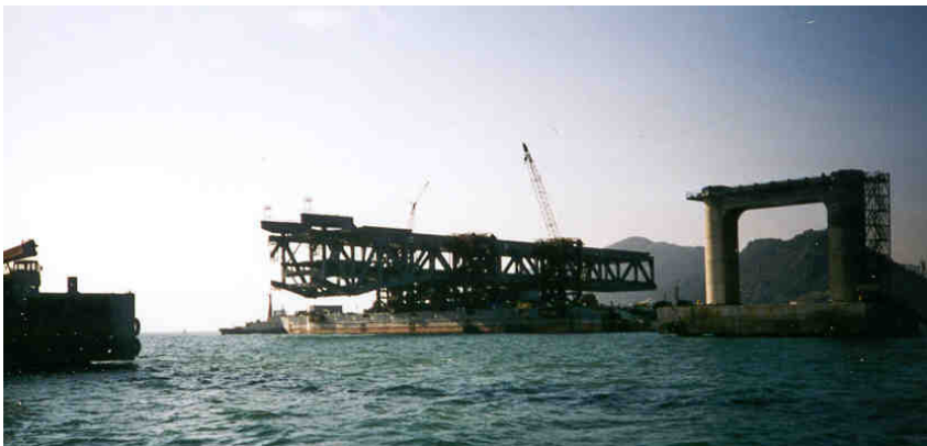
Kwang Ahn Bridge Span
